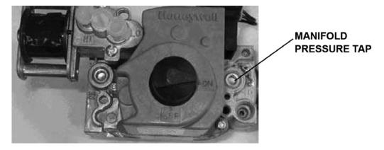
Figure 8. Gas Valve Manifold Pressure Tap
