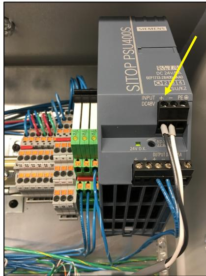
*CoolLinks Power Converter 48VDC Connections*
