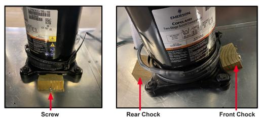
Figure 4 Compressor Chock Removal
