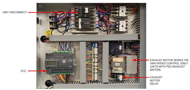
Figure 10. Electrical Control Box
