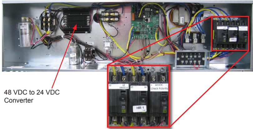
48 VDC to 24 VDC Converter
