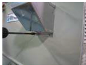
SECURE HOOD TO UNIT WITH TWO SCREWS
