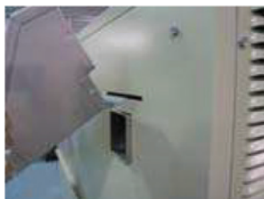
INSERT TAB IN THE HOOD INTO THE SLOT IN THE UNIT
