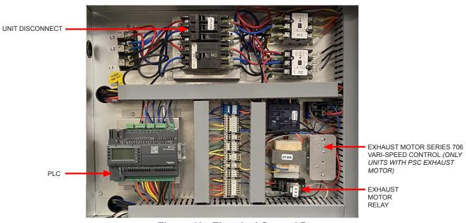
Figure 10. Electrical Control Box
