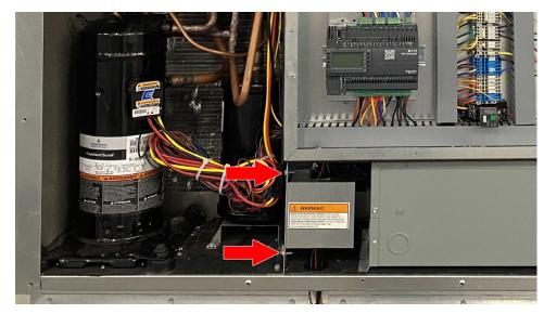
E. After removing the interior panel cover, disconnect the wiring to the blower assembly and the four wires to the transformer.
